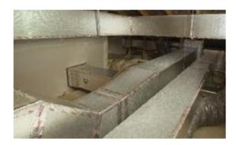
Traditionally, HVAC ductwork is constructed from galvanized sheet steel, which is installed first and then insulated separately as a second operation. The *Kingspan* **Kool**Duct® System however, is an advanced and innovative pre-insulated rectangular HVAC ductwork system, which is installed in a single-fix.
