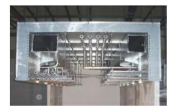
The low weight of ductwork fabricated from The *Kingspan* **Kool**Duct® System makes it especially suitable for use in pre–fabricated modules, which may have to be transported long distances to site. Moreover, the requirement for specialized heavy–duty mechanical handling and lifting equipment can be reduced, which makes ductwork fabricated from The *Kingspan* **Kool**Duct® System particularly favorable for riser sections that span multiple stories in high–rise buildings.
