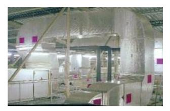
A key factor in the difference shown is in the cost of labor manhours. The construction, installation and insulation activity of the sheet steel ductwork system, accounted for 714.75 hours. In contrast, the fabrication and installation of ductwork from The *Kingspan* **Kool**Duct® System, only required 513.75 hours – providing a labor man–hour saving of 28%.
