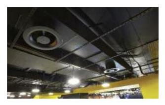
Ductwork fabricated from The Kingspan KoolDuct® System is the only premium performance pre-insulated ductwork in the world to be UL Listed as a Class 1 Air Duct, to Standard for Safety UL 181 (Underwriters Laboratories: Factory Made Air Ducts & Air Connectors), when fabricated to a specification clearly defined by UL.
