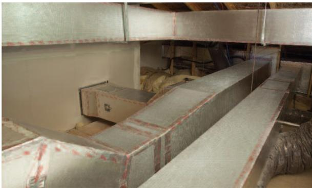
Traditionally, ductwork is constructed from galvanized sheet steel, which is installed first and then insulated separately as a second operation. The **Kingspan KoolDuct® System** however, is an advanced and innovative pre-insulated rectangular HVAC ductwork system, which is installed in a single-fix.
